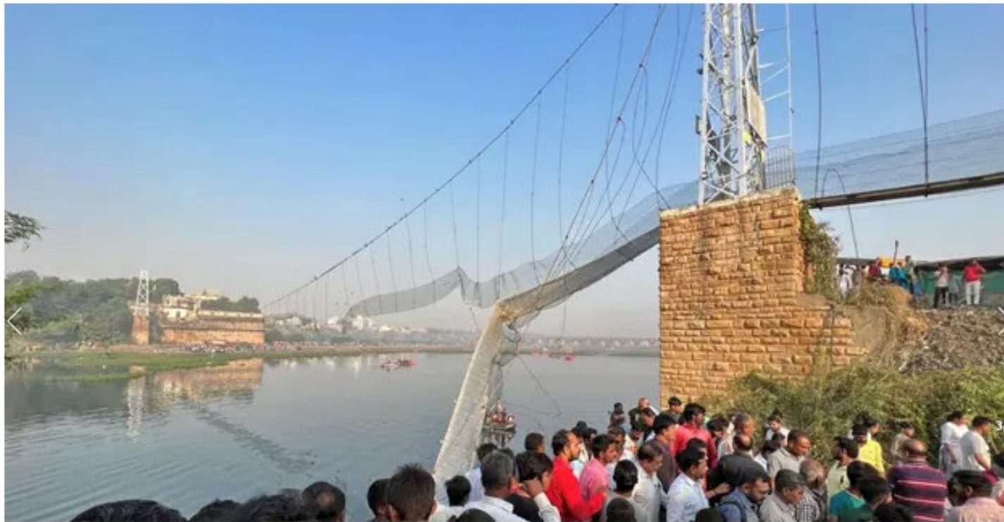
The morning after. Morbi pedestrian deck collapsed after suspension cable gave way.
